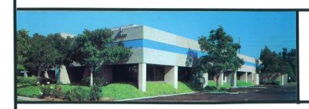
RIGGINS CONSTRUCTION & MANAGEMENT, INC. constructed a 33,235-SF single story industrial/office facility having 75 percent office capability and 25 percent light industrial use. The facility was designed to accommodated two tenants and was constructed utilizing concrete tilt-up methods featuring ribbed concrete panels which accented the buildings attractive entries.
